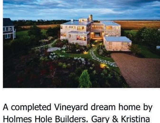
A completed Vineyard dream home by Holmes Hole Builders. Gary & Kristina started Holmes Hole Builders 20 years ago, previously involved in wooden boat restoration and sailing.
